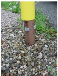
**Step Two** – Install Bollardgard over Gripper Tabs. Gripper Tabs should provide a tight installation which cannot be easily removed.
